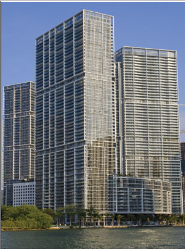
ICON Brickell includes two 57-story residential towers and a third condominium tower 50 stories high that also includes a hotel component. (Photo by Smith Aerial Visions/ www.smithaerial.com )
